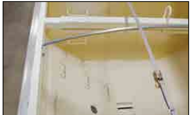
Fig 30 - Compartment ladder rungs
