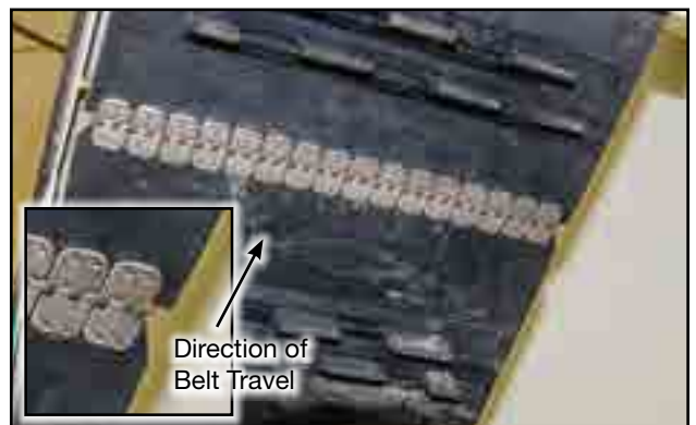
Fig 71 - Alligator lacing on rear conveyor paddle belt
